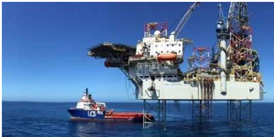
Noble Tom Prosser Drilling Rig during the Caley well test
